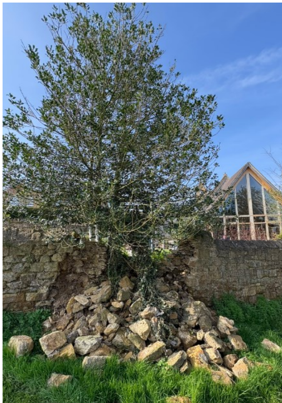
Collapsed wall to be repaired after removal
