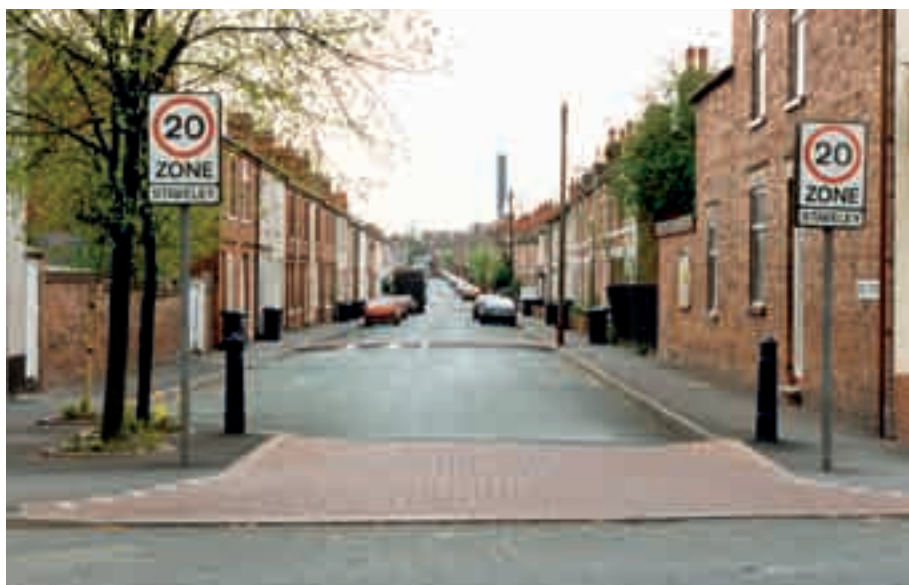
Fig. 7.2 Entry treatment at the start of a 20 mph zone
